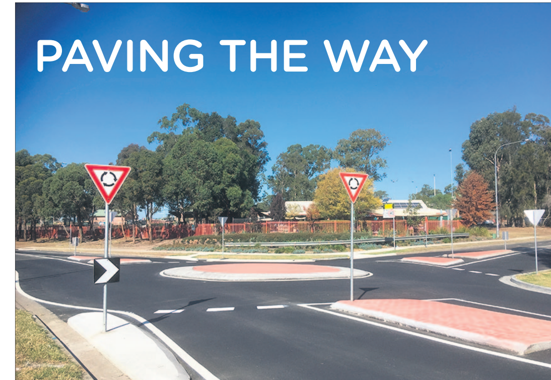
This roundabout in Erskine Park is one recent improvement
