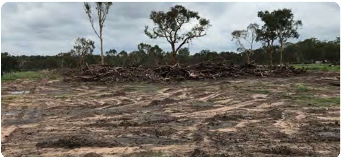
Figure 41. Land clearing at Castlereagh (Penrith City Council 2025)
