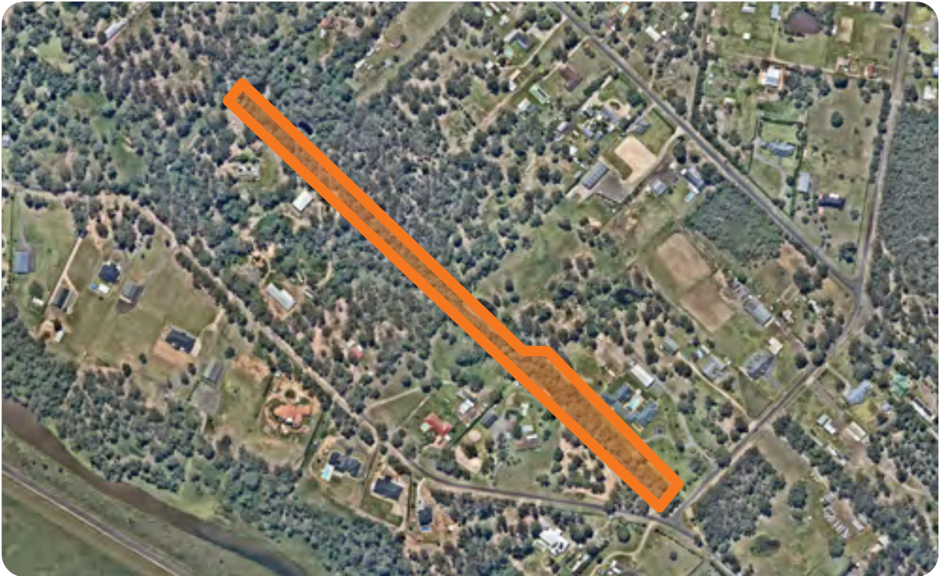
Figure 51. Tempest Street aerial imagery (Nearmap 2025)
