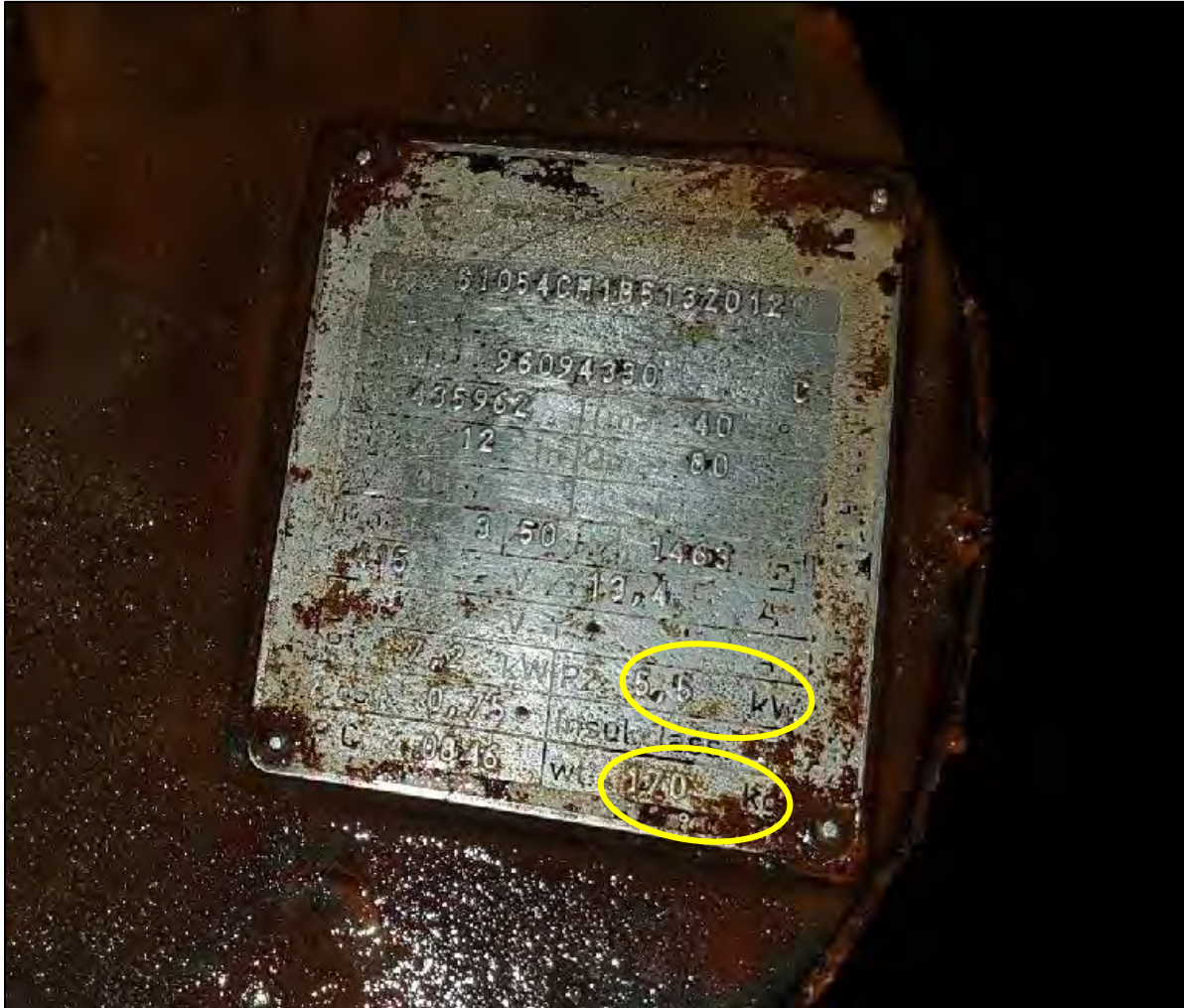
Plate 6 Identification Tags for Pump #1
