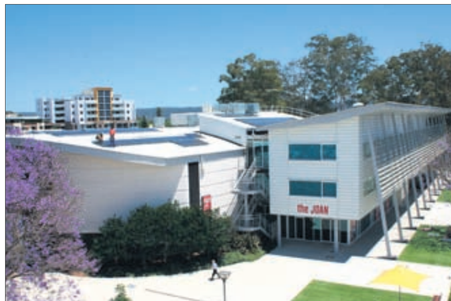
Council has installed 34 solar panel systems on our facilities, including the Joan.
