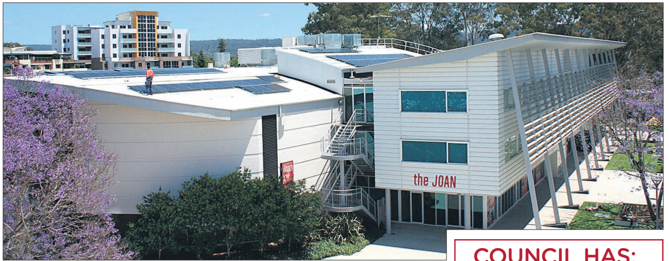
Solar panel installation on the Joan Sutherland Performing Arts Centre
