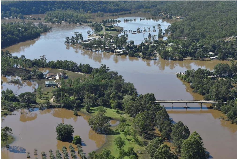
Figure 5-31. View of the Colo River Junction (looking from the Colo River) – 26 March 2021 (Source: Infrastructure NSW. Photo: Adam Hollingworth)
