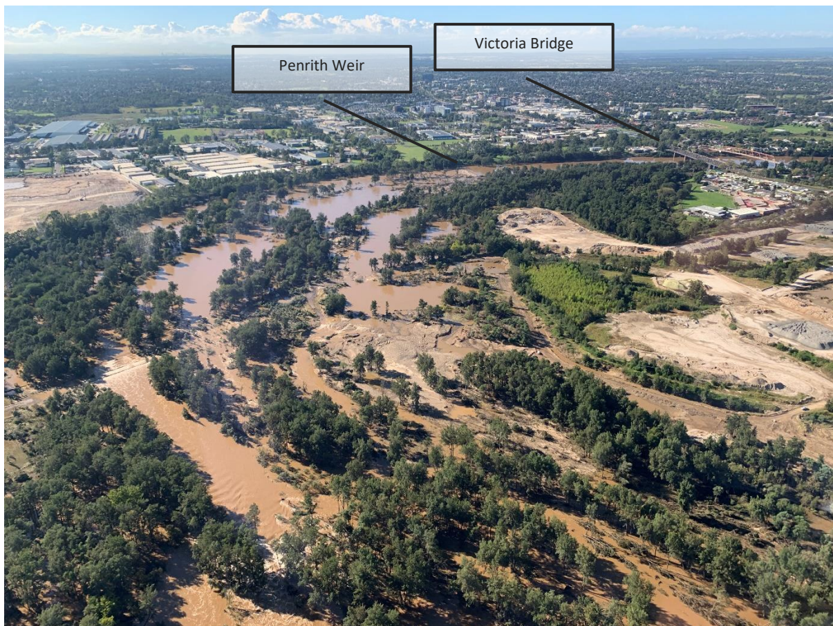
Figure 5-9. View from downstream looking toward Victoria Bridge and Penrith Weir (26 March 2021)
