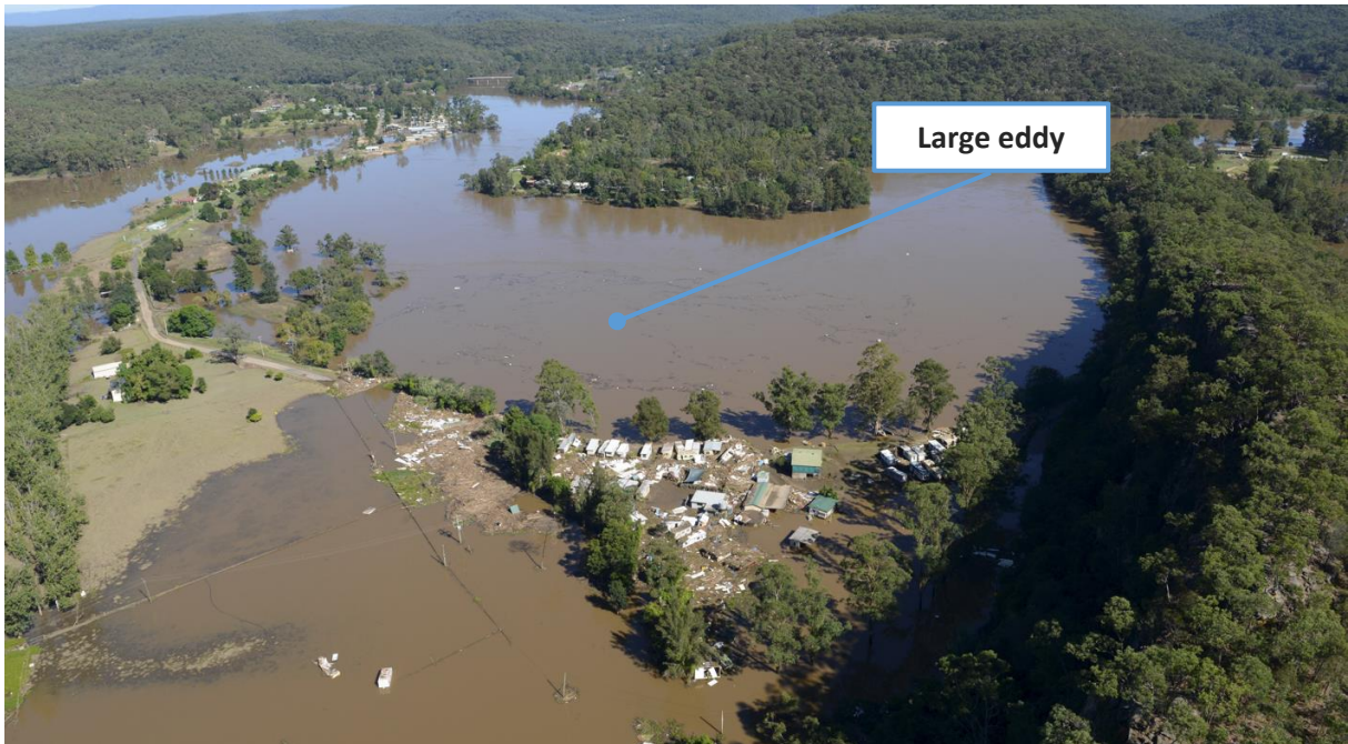
Figure 5-36. Oblique View of St George Caravan Park and Large Eddy (26 March 2021, Source: Adam Hollingworth)
