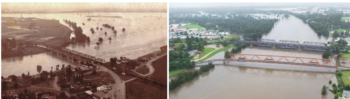
Figure 5-18. View of Flooding Downstream of Victoria Bridge (left : 1961 13 , right : 2021 14 )
