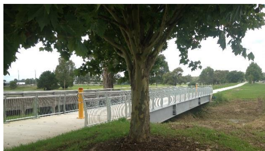
Figure 8 Shared Path Bridge over Surveyors Creek in Jamison Rd, Jamisontown
