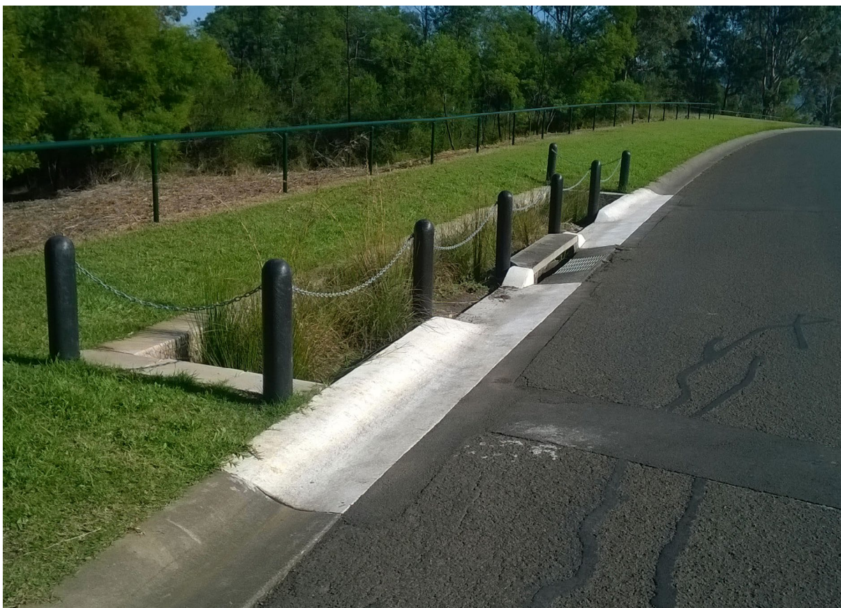
Soling Crescent Raingarden.
