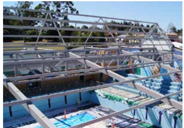
» RIPPLES ROOF REFURBISHMENT
