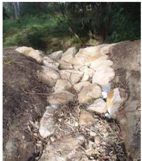
▲ Use of rocks to stabilise the bank and reduce erosion at Werrington Creek.
