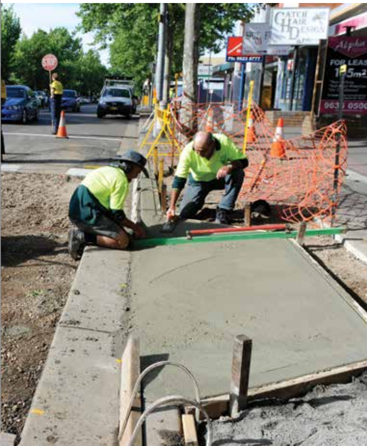
▲ Shared pathway construction.
