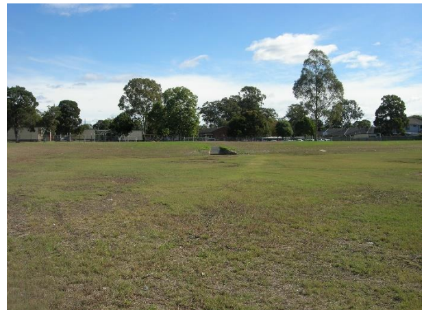
Photo 21: Oxley Park basin outlet and spillway
