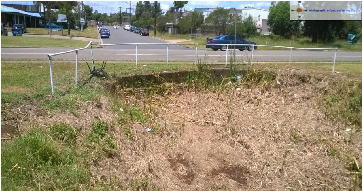
Photo 9: Outlet of pipe at Kurrajong Road near Plasser Crescent
