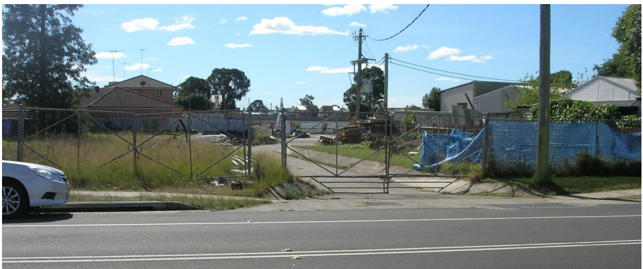
Photo 11: Overland flow path at 77 Carpenter Street (surcharge grate in foreground)
