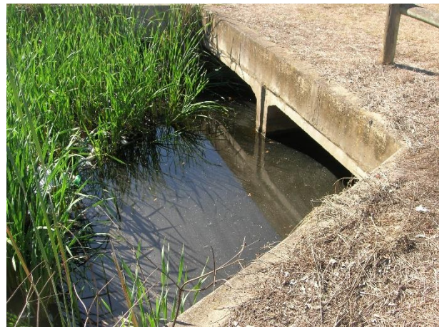
Photo 15: Primary trunk drain outlet at Kurrajong Rd showing stagnant water
