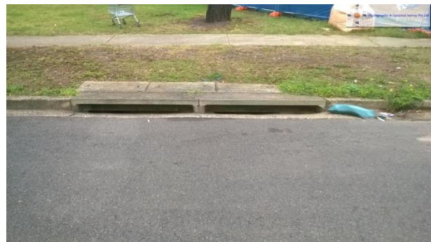
Photo 14: Drainage pit along Hobart Street
