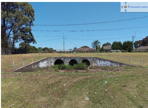
Photo 25: Outlet from GWH cross-drainage pipes
