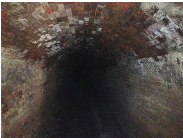
Photo 2: Brick arch culvert under railway
