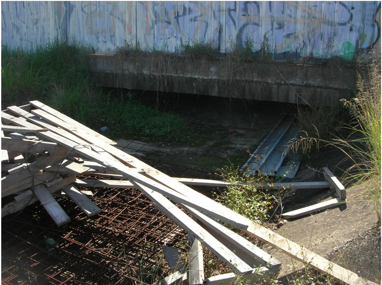
Photo 12: Covered open channel inlet under 4A Sykes Street from 77 Carpenter Street
