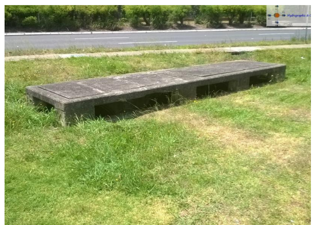
Photo 26: Inlet to GWH cross-drainage pipes
