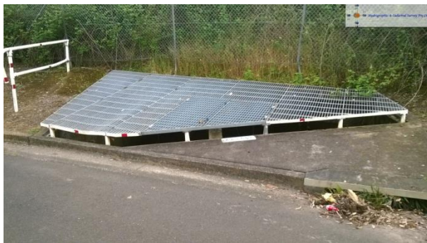
Photo 13: Trunk drain inlet on Hobart Street
