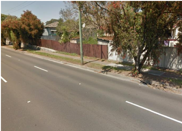
Photo 27: GWH low point (upstream side)
