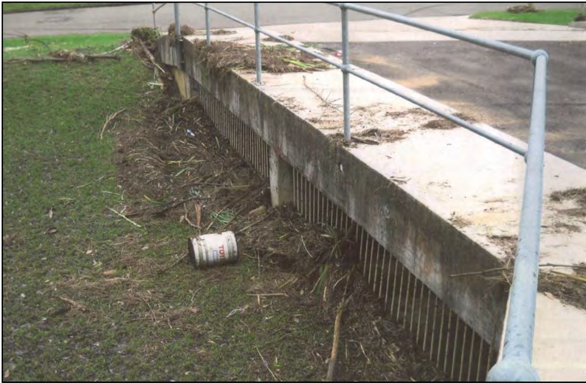
Plate 6 View showing debris accumulation upstream of Cosgrove Crescent culvert following February 2012 flood
