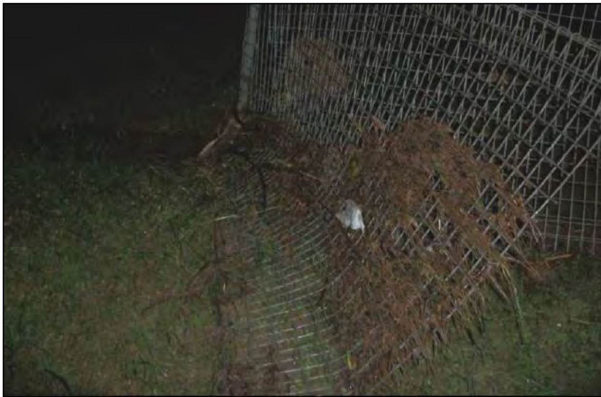
Plate 10 Collapsed fence adjoining Second Avenue, Kingswood showing debris mark approximately 0.5 m high (February 2012 flood)
