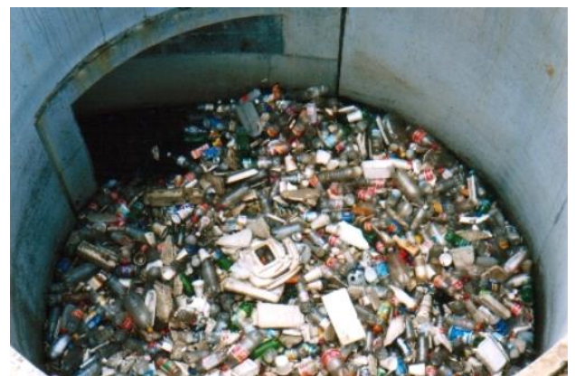
Image: Litter being capture by a Gross Pollutant Trap (GPT).
