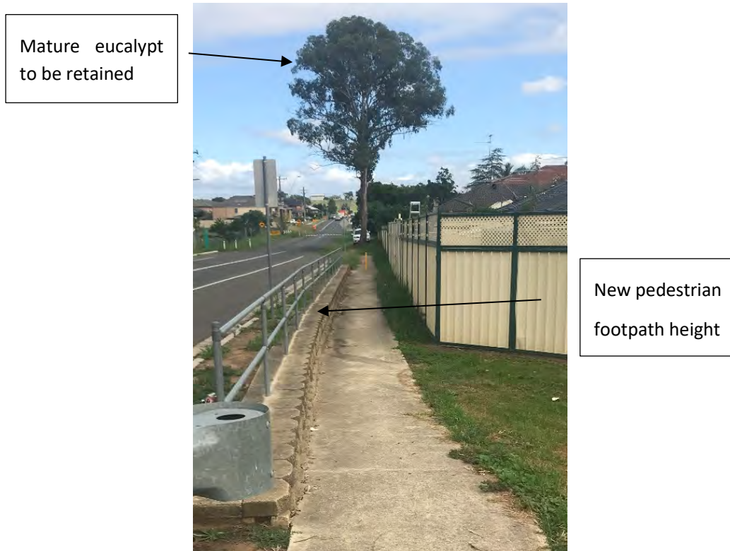
Plate 6. Large mature eucalypt that will be retained as part of the proposed works. The newly constructed shared footpath will be raised to the existing retaining wall height and will travel south around the root system.
