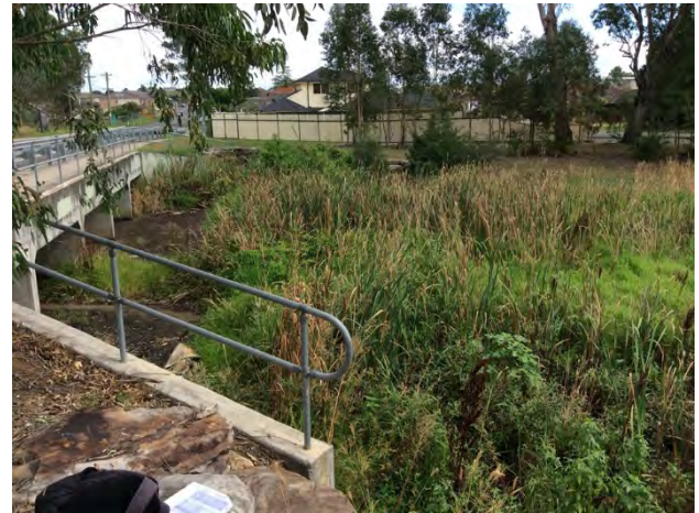
Figure 5-5 Claremont Creek crossing north of the culvert, showing emergent aquatic vegetation.
