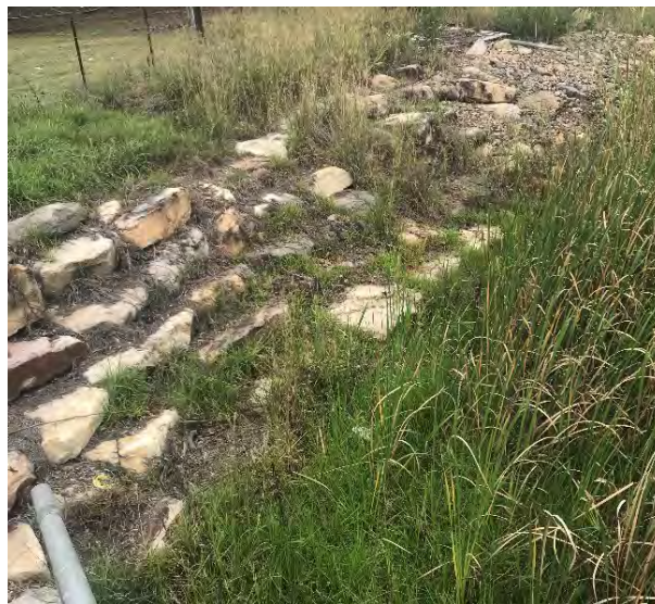
Plate 2. Claremont Creek bank modifications on southern side, facing southeast.
