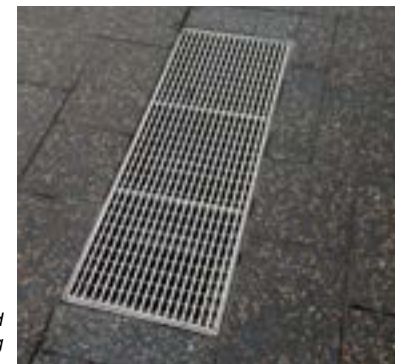
Stormwater cover installed square to paving
