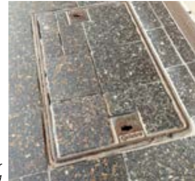
Infill service cover with unit paving
