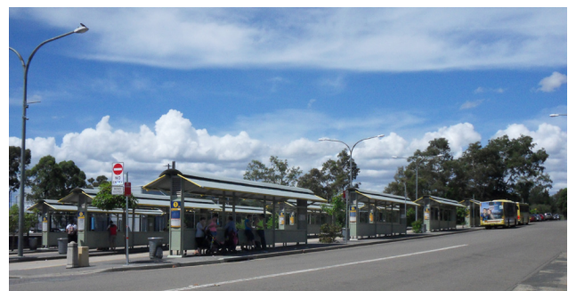
St Marys bus interchange, on Station Street at the northern end of Queen Street
