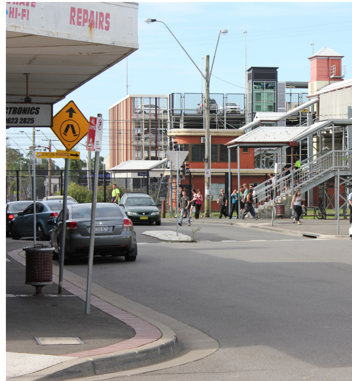
Configuration of pick up and drop off area at St Mary Square.
