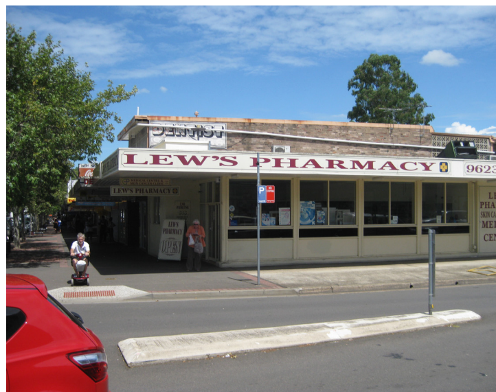
Transition of footpath area just west of Queen Street.
