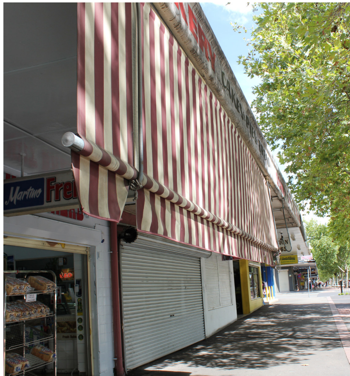
Footpath shading from afternoon sun exposure along footpath.
