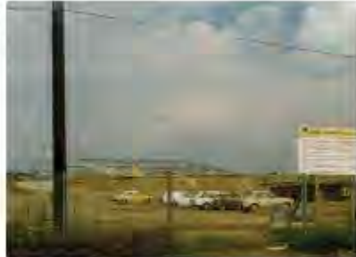
1986 TAFE NSW - Western Sydney Institute, Nepean College, Kingswood Campus under construction
