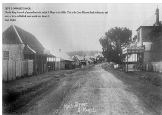
The Western Highway in the late nineteenth century. This is a streetscape characterized by the rows of freestanding buildings erected over about 50 years. The width of the road is quite narrow, but there is a generous margin to each side. Source: Stacker, L., Pictorial History: Penrith and St Marys , Alexandria, Kingsclear Books, 2002, p.110
