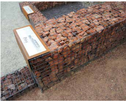
Gabion cages for brick interpretation Image credit: MUSEscape 2014
