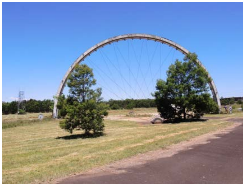
Figure 28 The steel and timber antenna hoop at the former Naval Radar Calibration Range. The figures at right indicate the large scale of this structure. An associated tower is visible in the background at left. (Photo: Chris Betteridge, 18 November 2014)
