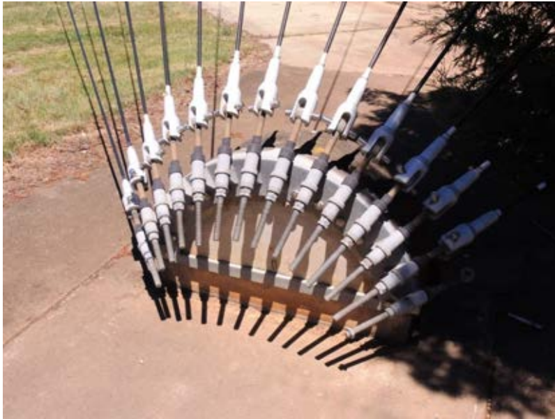
Figure 29 One of two structures holding the supporting cables for the hoop antenna. (Photo: Chris Betteridge, 18 November 2014)
