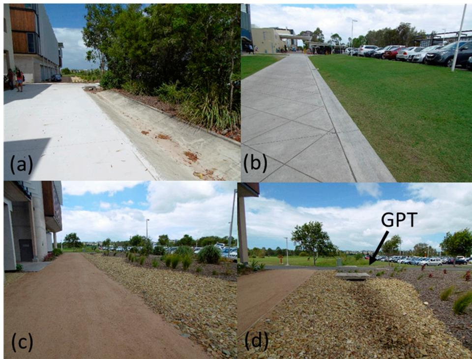
**Figure 3.** Catchment characteristics: (a) concrete surfaces; (b) carparks and grassy slopes; (c) rock swales; and (d) pit entry to underground pipe (arrow shows GPT location).
